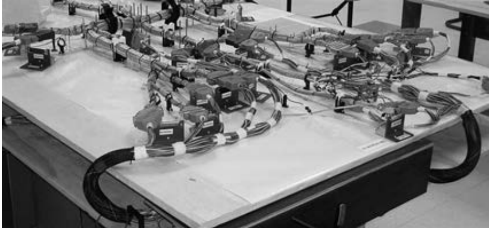
Galaxy Wire & Cable does 100 percent continuity testing.
