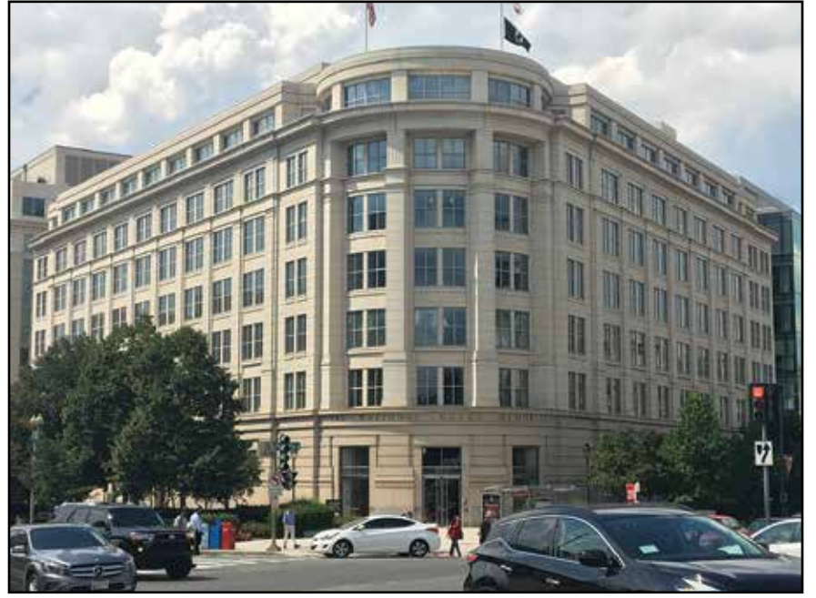
Amtrak's New Headquarters in Washington, D.C
